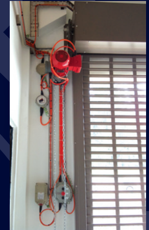
Panorama Vision Shutter with Explosion-proof motor & fittings (EXD Class 1 Zone 1)
